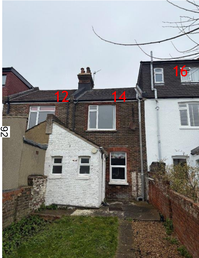
Fig 2.0 Photo of existing rear elevation of application site
