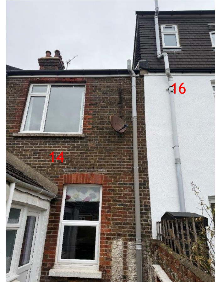
Fig 2.3 Photo of existing rear extension of the application site
