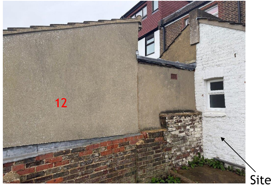
Fig 2.1 Photo of existing rear extension and neighbouring extension at no. 12
